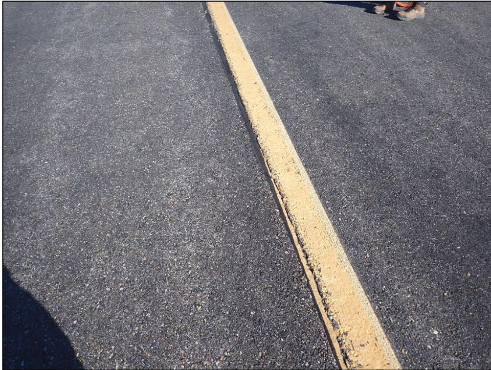
TW-01-05: L&T Cracking
