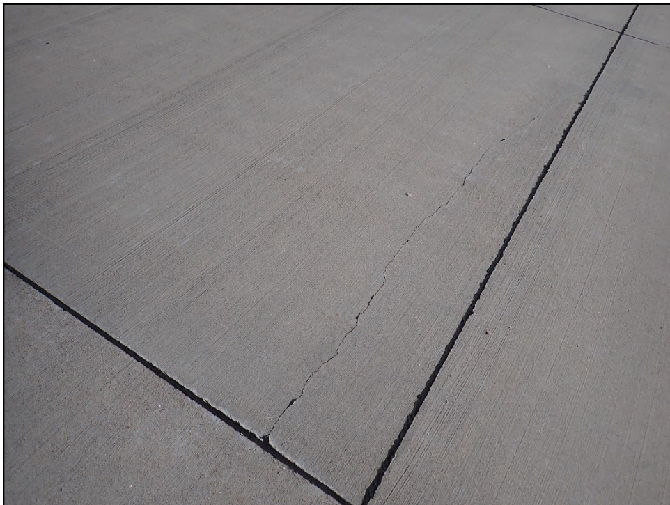
AP-03-02: LTD Cracking
