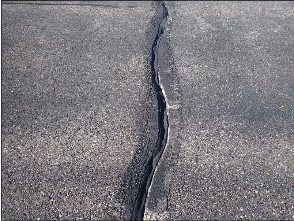
RW08-01-47: L&T Cracking
